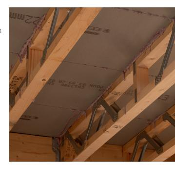
It is essential that the boards are fitted correctly to the joist, the joint is secure (bead of adhesive in the groove and shoulder of the tongue), and that glue is forced up and out of the top surface joint (shoulder of the tongue). The bead of glue applied in the groove of the board will firmly hold the joint in place and will expand out below the joint to protect the underside of the board from moisture ingress.
